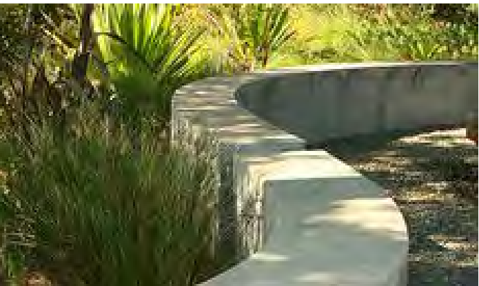
13. Concrete retaining wall
