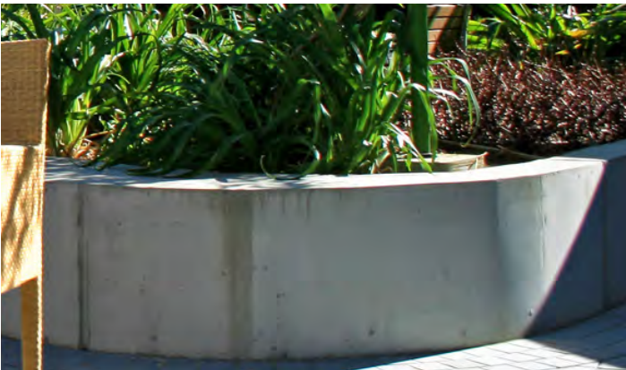
21. Raised Concrete Planter
